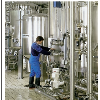
Food processing plant
