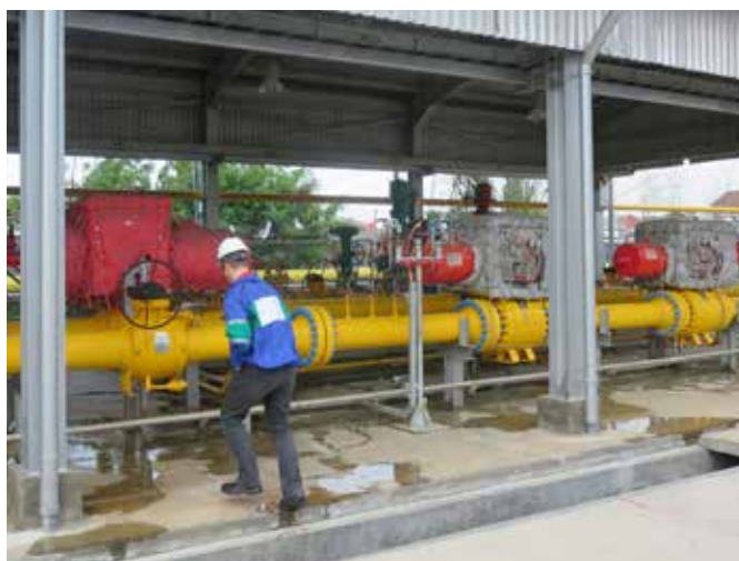
Construction of gas pipeline for Kalimantan Jawa Gas, Indonesia
